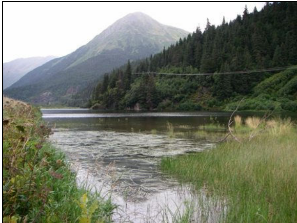
Photo 1. Surface water impounded by the highway may have the capacity to recharge groundwater.
