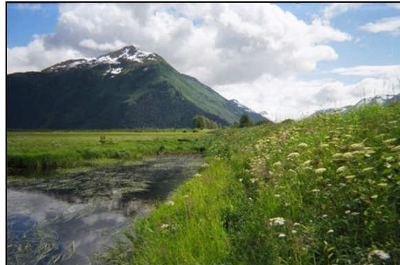
Photo 5. A typical vegetated road embankment along the Seward Highway abutting a flooded wetland.
